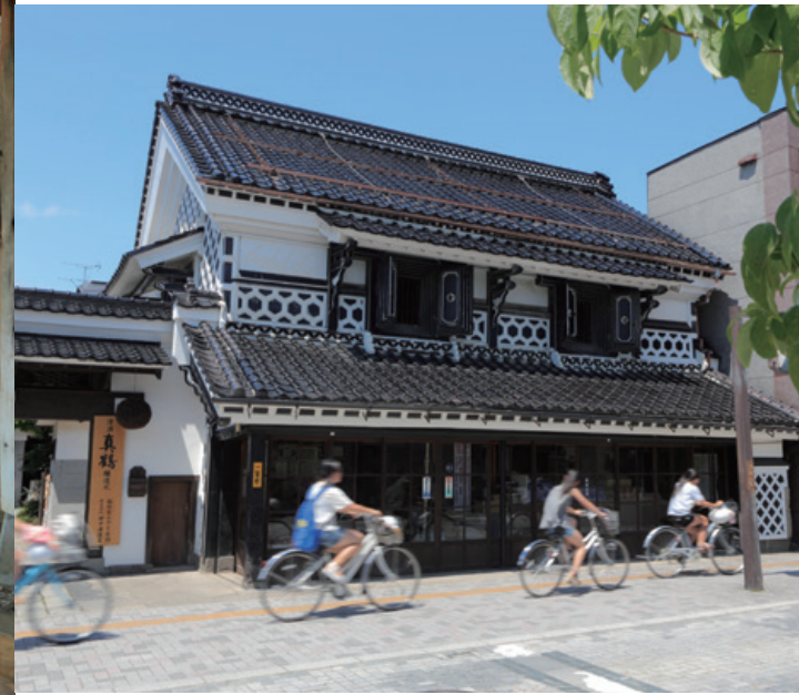
This unusual building has black and white namako-kabe (walls covered with square tiles jointed with raised plaster).
